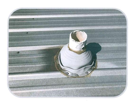
DESCRIPTION OF DEFICIENCIES: Deteriorated flashing at pipe penetrations.
