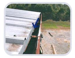
DESCRIPTION OF DEFICIENCIES: Surface rust at curb, rake edge and gutter Approx. 600 feet
