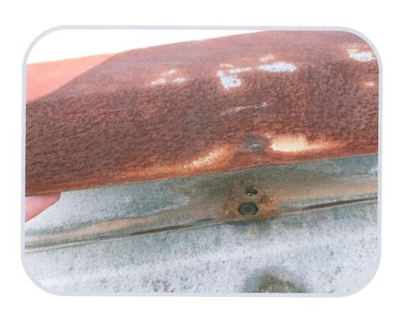
DESCRIPTION OF DEFICIENCIES: Rake edge is missing butyl tape and fasteners Approx. 180 feet
