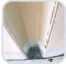
DESCRIPTION OF DEFICIENCIES: Improper roof to wall installation Approx. 85 feet
