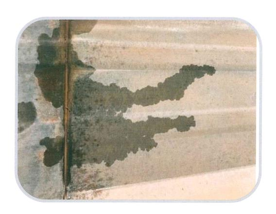
DESCRIPTION OF DEFICIENCIES: Sealant at field seams starting fail Approx. 400 feet
