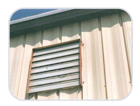
DESCRIPTION OF DEFICIENCIES: Sealant around vents starting to fail 4 each
