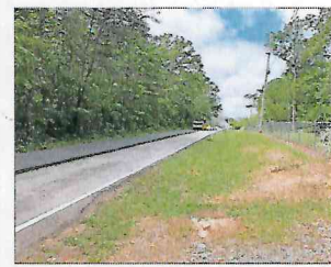
Officials say pavement failures will be repaired before the final layer of paving on Hog Jowl Road.
