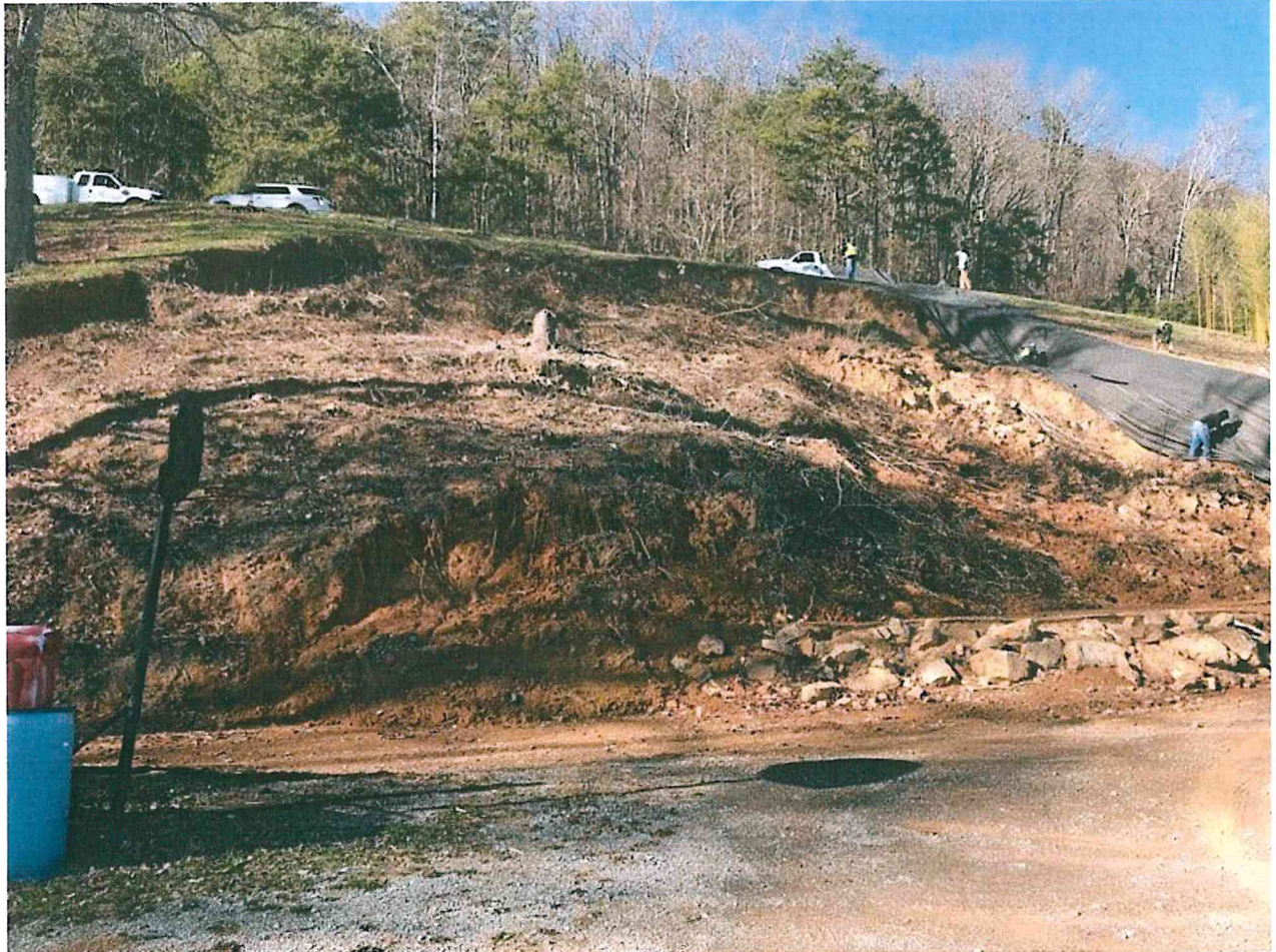
Photo 2: Previous slope failure to the west of the current landslide (recent landslide is to the right)
