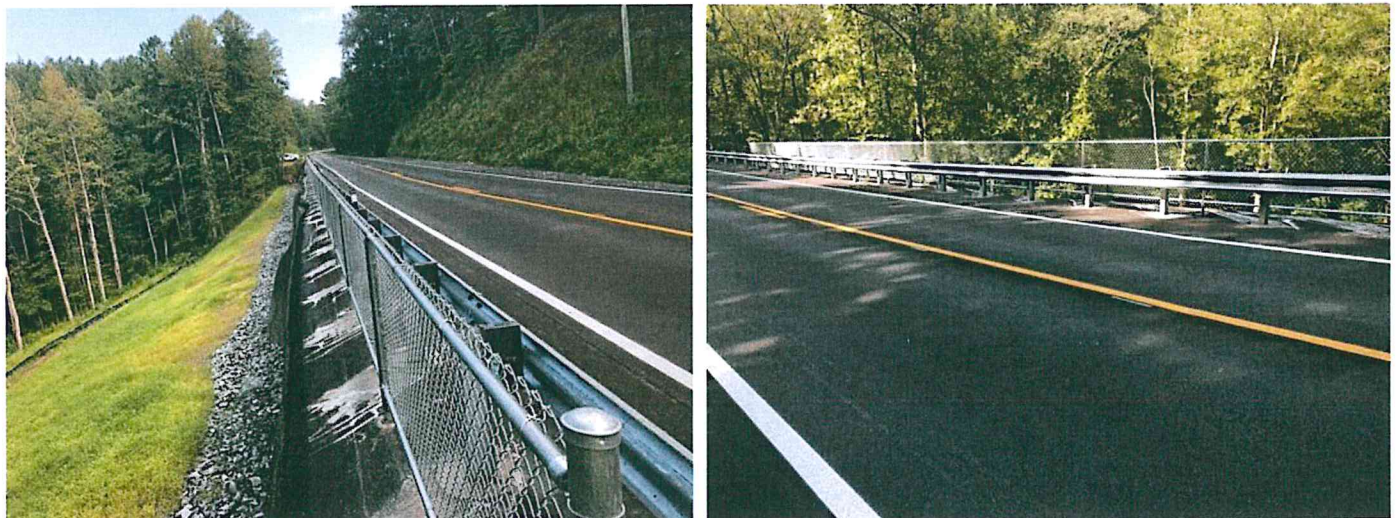
Photo 6: Finished photos of similar Pickens County GA project showing guardrail and safety fence
