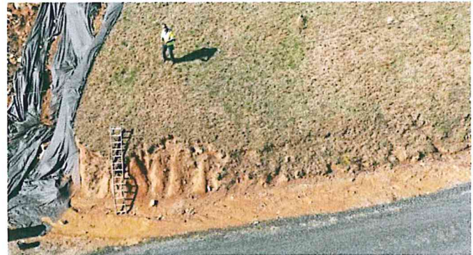
Photo 3: Toe of slope condition left and right of recent landslide
