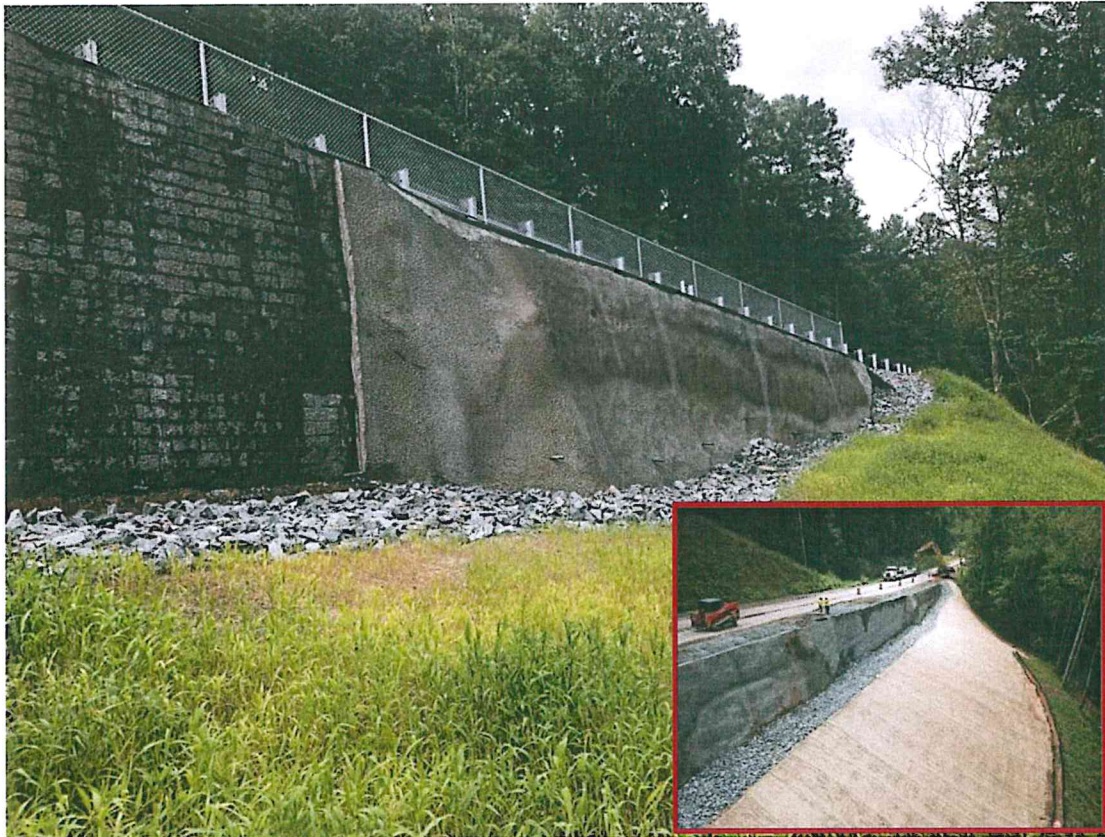
Photo 5: Similar Pickens County GA project with Soil Nail and GSC Walls
