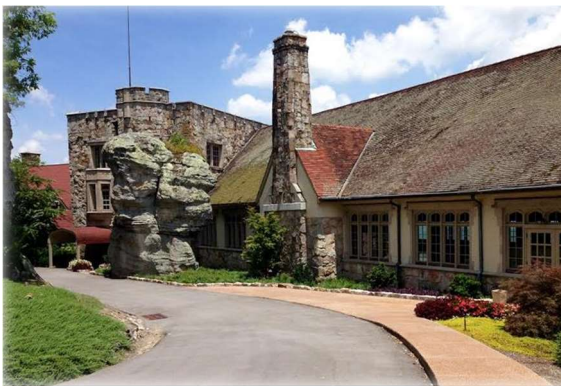
Figure 13. Lookout Mountain Club - https://lookoutmountain.club/home
